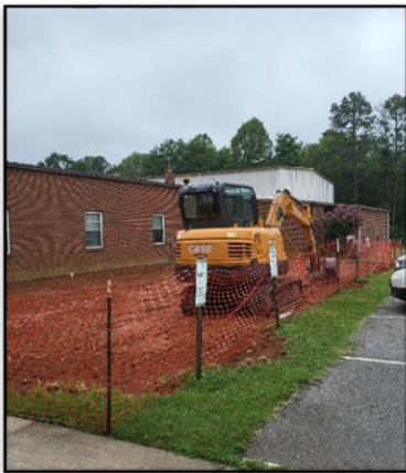
2026 Drainage Project in-progress!
