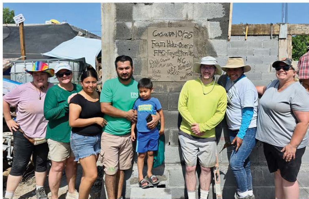
FPC's Mexico Mission Team with the Hernandez Osorio Family standing by the newly built walls of Casa #10 in 2025.
