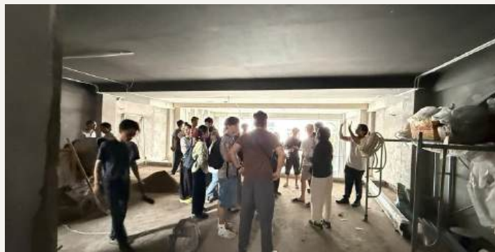
AMI Center Building Progress
