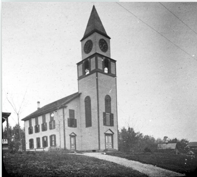
Parker, W. S. (ca. 1870-1930). "Methodist Episcopal Church." The church was built in Quincy, Florida. https://www.digitalcommonwealth.org/search/
