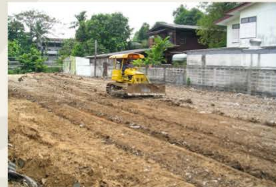
Land next to the khlong.
