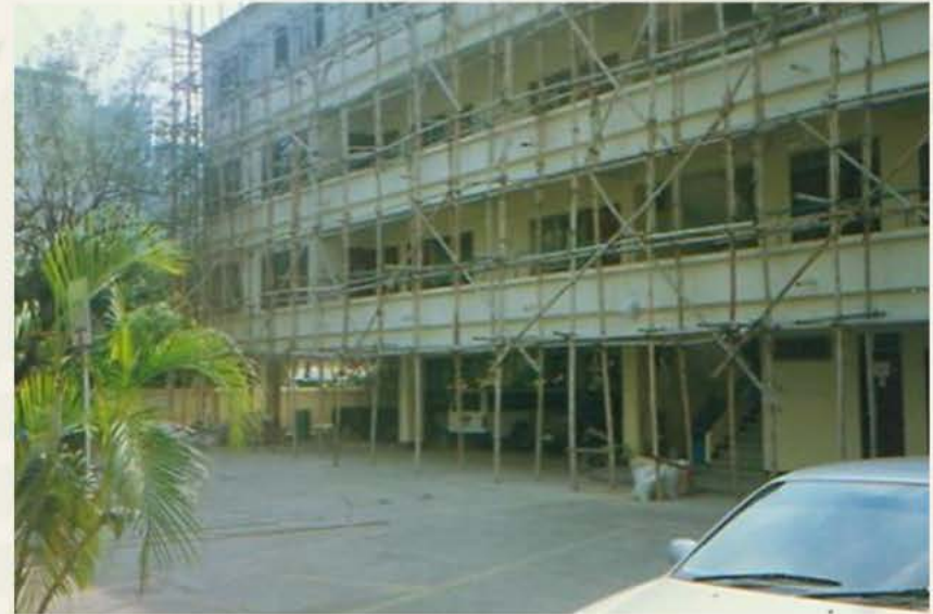
Adding a fourth floor to the education building.
