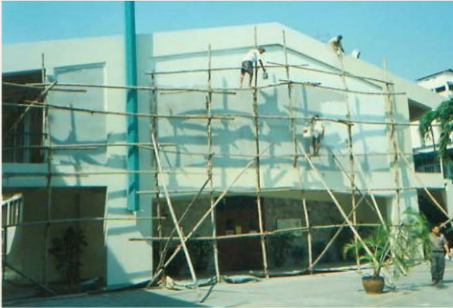
Building an extension to the sanctuary.
