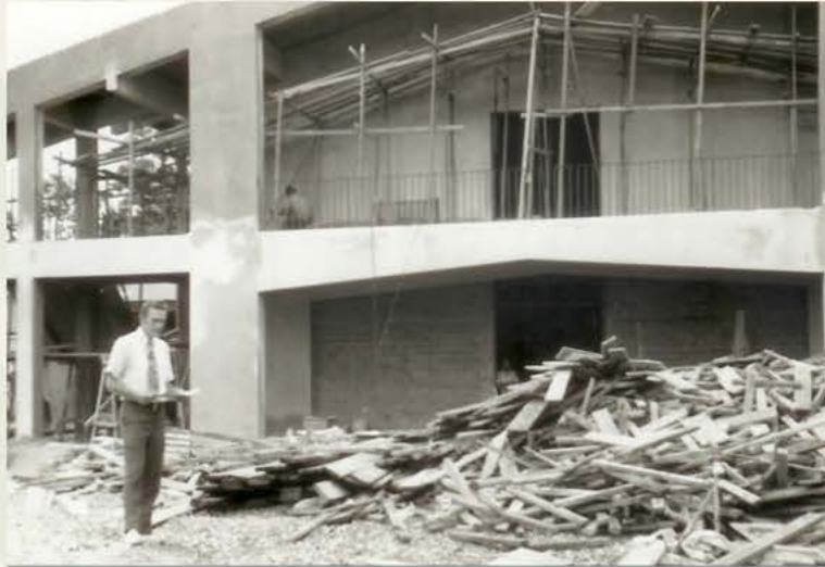
Construction of the sanctuary at 42 Sukhumvit 10.
