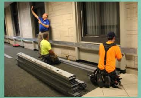
Structure preserving Martin Hall wall: John Meek and Felmley Dickerson Construction
