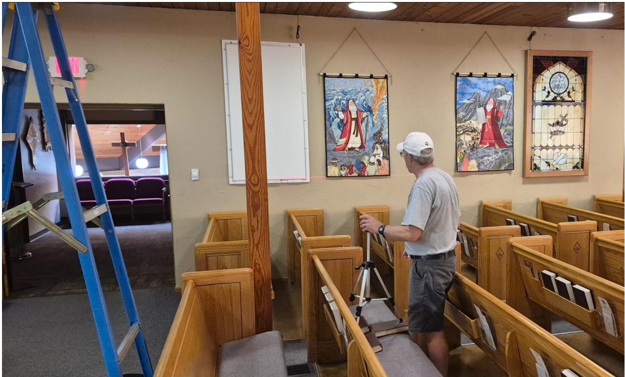
Ken Paul during installation of the frames
