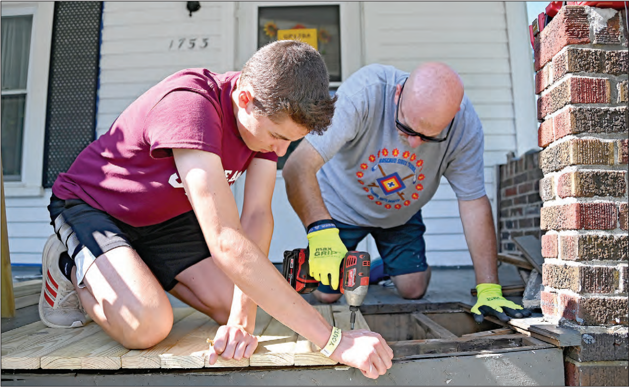
Matt Cassidy and Will Huber put new boards over a hole in a front porch on Roslyn during the Workcamp visit in 2024.
