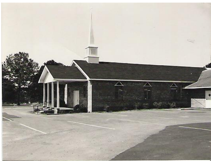
Brick Church Building
