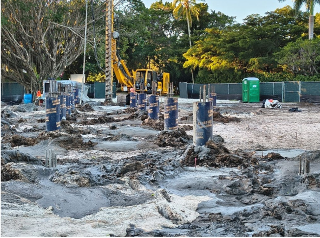
Auger cast piles forming a deep foundation. The taller piles mark the location of the nave.
