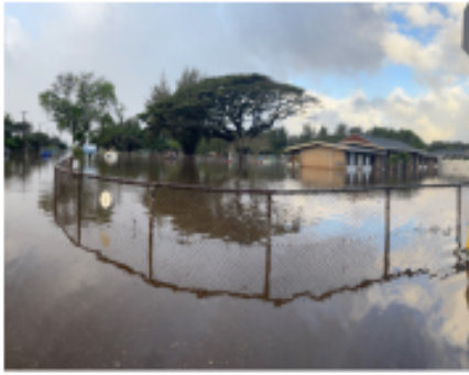
Floods at the church in Haleiwa.
