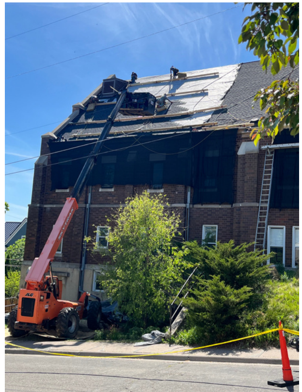
Construction at the St. Anthony Park Campus that was completed in June of 2026
