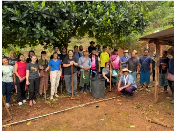
Eastside Team Connecting PVC Water Pipeline to Village Homes
