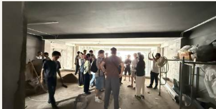
AMI Center Building Progress
