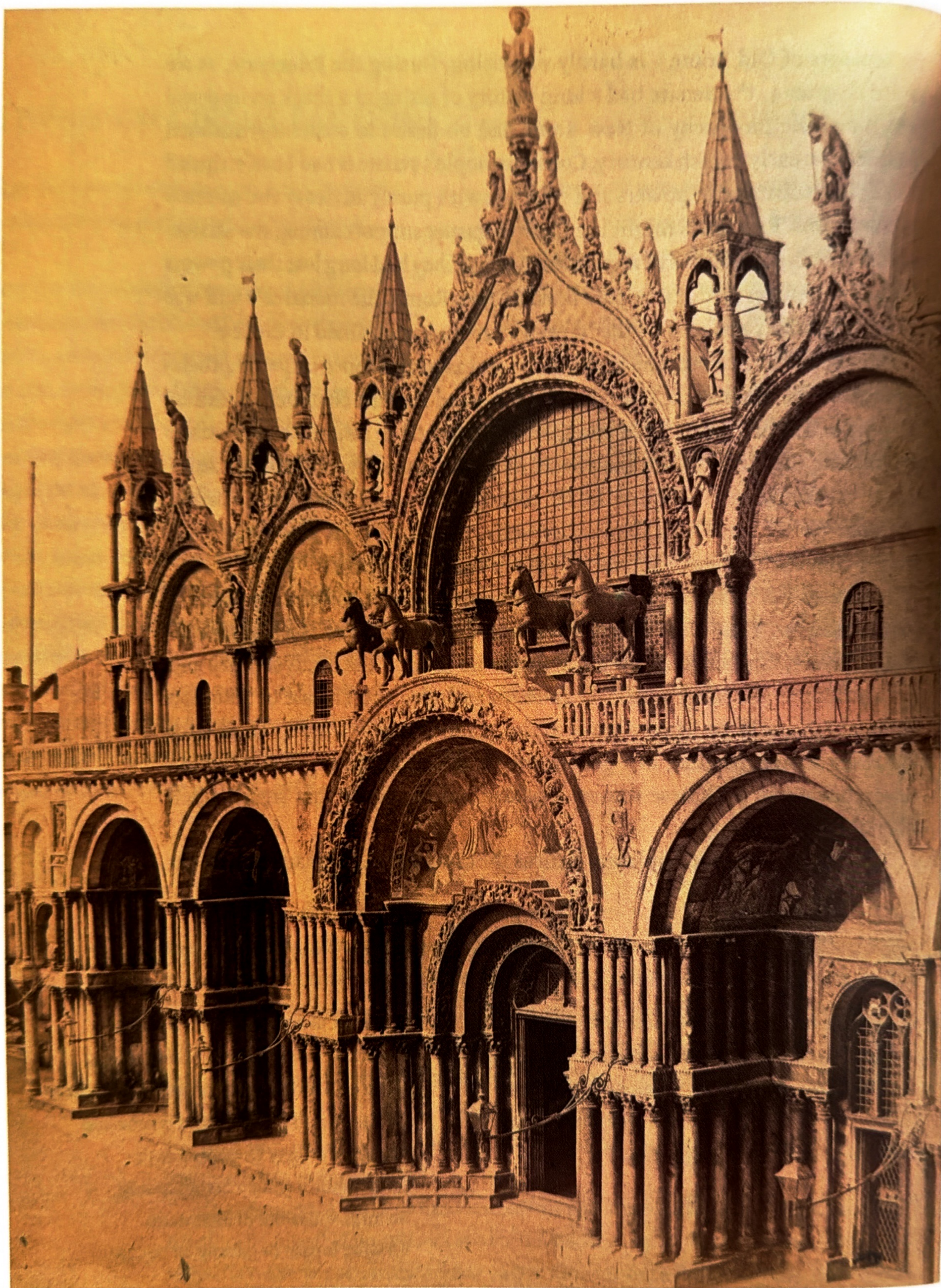
FIGURE 6.10. Principal facade of St. Mark's Basilica in Venice, Carlo Ponti, circa 1860–70. Here the original horses can be seen as placed on the loggia .
